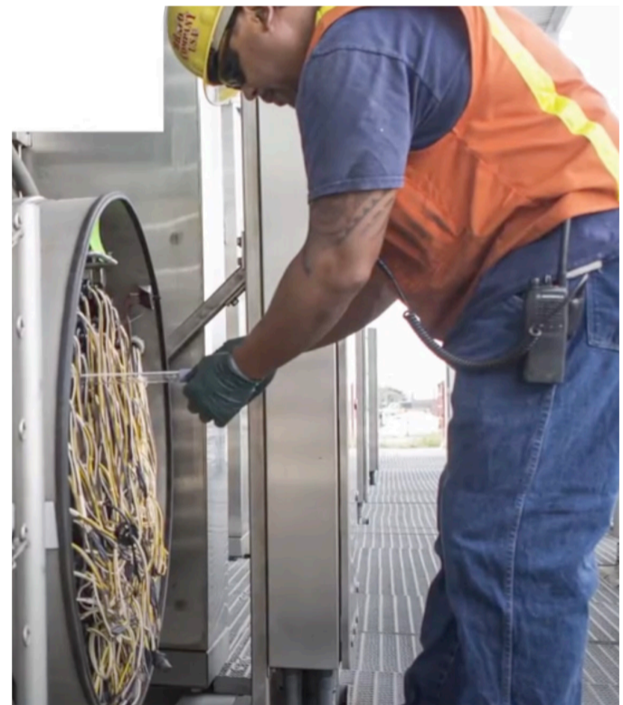
Image: Orange County in southern California has built a 500-million-dollar state-of-the-art water treatment plant which turns raw sewage into pure drinking water. The biggest challenge for the authorities is not the technology but selling the public on the process known as from toilet-to-tap.
