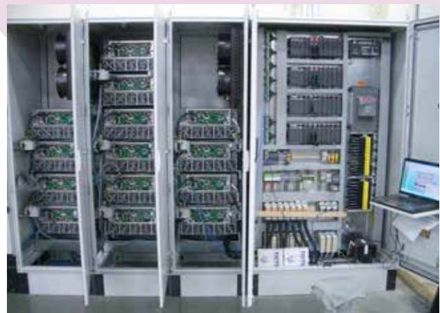
▲ Situation after installing Nedap UV lamp drivers
